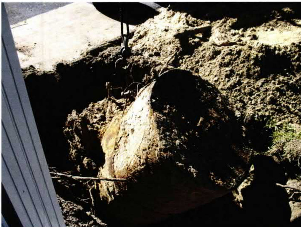
Picture 2: UST 367Aspen removal in progress.
